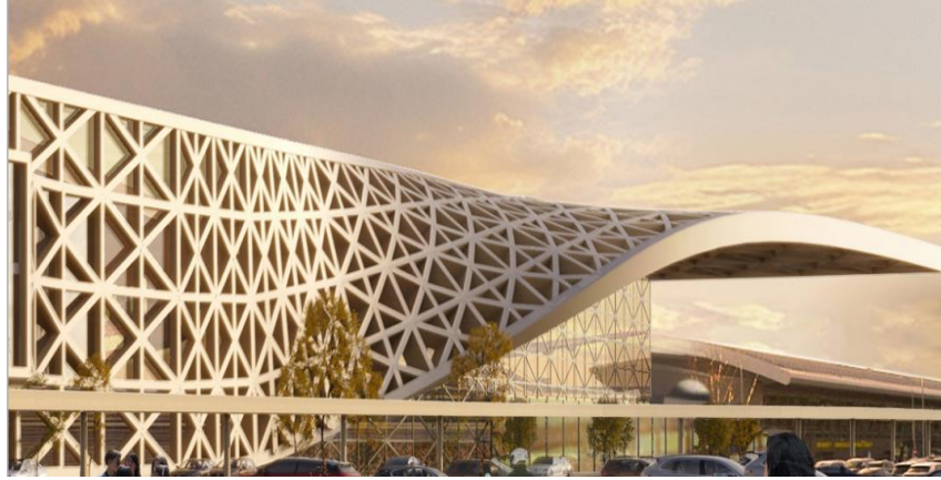
Fig. 4. Adaptive color effects achieved through the use of metal-ceramic panels (“QUANTUM CERAMIC”) and aluminum panels with an internal honeycomb core (“QUANTUM PARUS”). The façade changes its hue depending on the time of day, weather conditions, and the angle of sunlight
