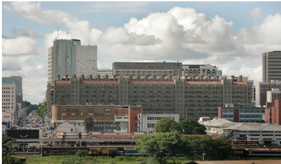
Pic. 2. The passive cooling design of the Eastgate Centre in Zimbabwe, with its distinctive chimneys, was inspired by termite mounds.
