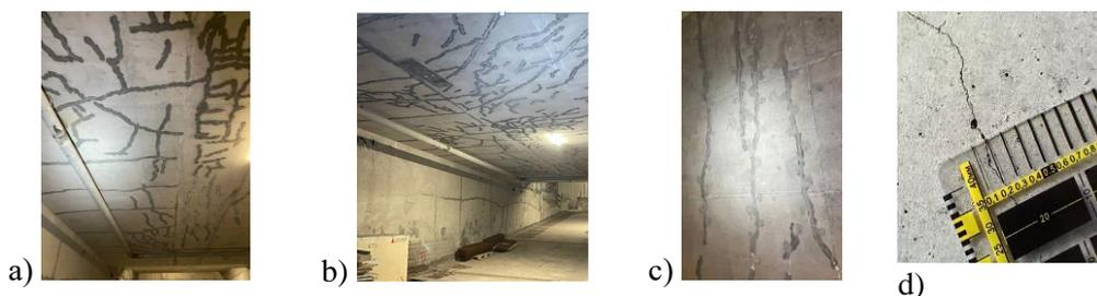
**Fig. 6.** Cracks detected during the inspection: a - in the floor slab of the 1st floor, b - in the floor slab of the 2nd floor; c - in the exterior walls of the underground -2nd floor; d - measurement of the crack width (0.2 mm).
