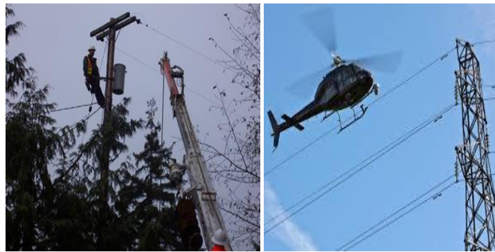
Figure 1(a). Ground inspection Figure 1(b). Aerial inspection
