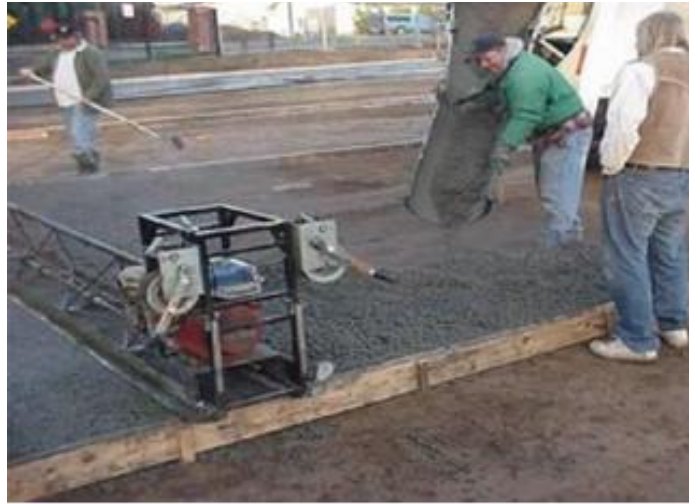
Figure 4: Finishing Of Pervious Concrete
