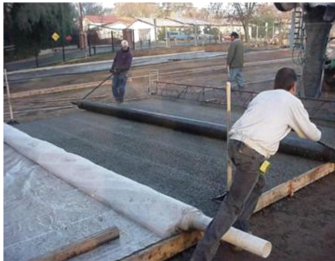
Figure 5: Compaction of Pervious Concrete
